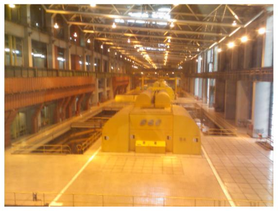
This picture shows some of the generator in the power station. There are altogether eight generators. As electricity cannot be stored, some of the generators will be turned off at night, when there is a time the demand of electricity is not very high, to reduce the energy loss. To turn on the generator again, it takes only an hour, which is convenient.
