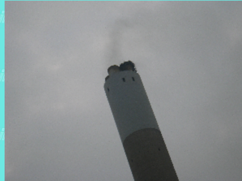
The smoke come out from the furance
