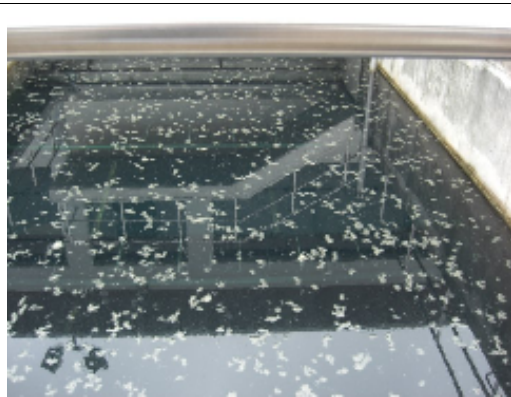
Alum is added to allow impurities in water to form a larger particle
