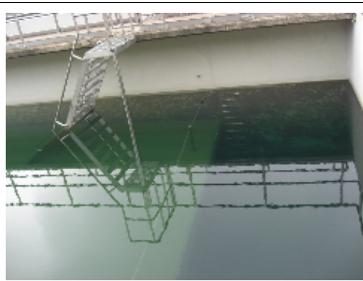
It is then pass to flocculation tank. larger particles are then coagulated.
