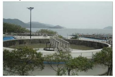
In primary sedimentation tanks, about 50% of the suspended solids in the preliminarily treated sewage are settled out and removed as primary sludge by sludge scraping mechanisms.
