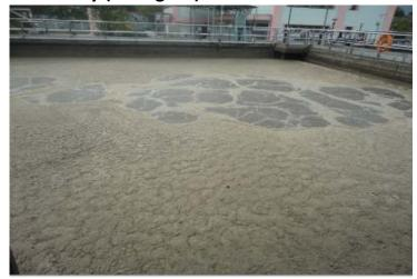
This is a Secondary (Biological) Treatment. In aeration tanks, compressed air is fed continuously to provide oxygen essential to sustain the growth of micro-organisms (activated sludge), which will assimilate pollutants in the sewage. The reaction time is about 6 hours.
