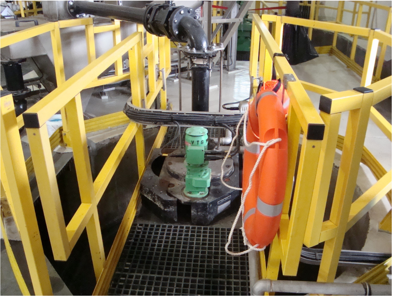
This is a process that can remove the oil with air flotation equipment from the sewage in the tank so as to further clean the sewage.
