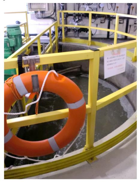
This is an area where it separates oil and the polluted water. As the area is dangerous, if a person fall into the tank, he will be drowned. Therefore, safety is very important.
