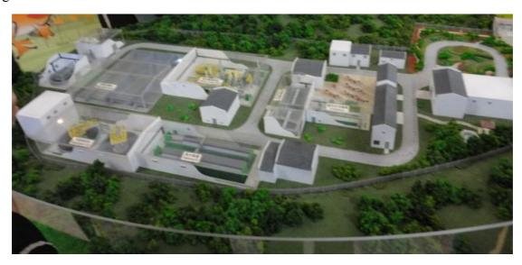
The modal in the photo shows the facility in the Ngong Ping Sewage Treatment Works. Preliminary treatment work, sequencing batch reactor and dual media filter are the three main processes.
