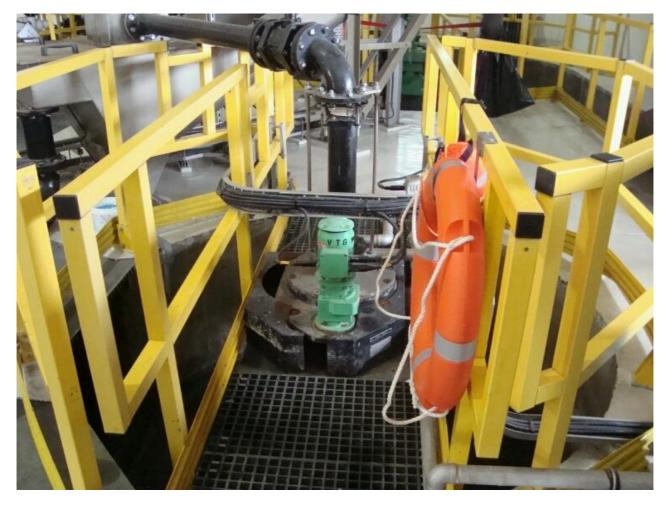
This is the Vortex Grit Trap. Its turbine moves slowly to separate large solids, grease and grit from the sewage in order to protect the downstream treatment process.
