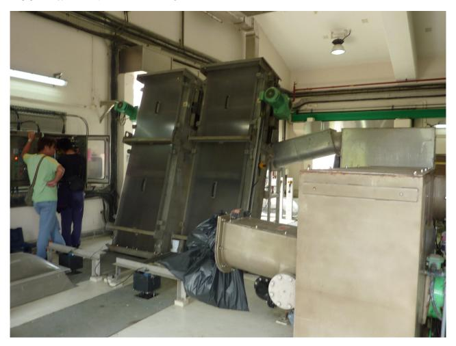
This machine is used to press the solid waste in order to take out the water in the waste and make it ready for other process.
