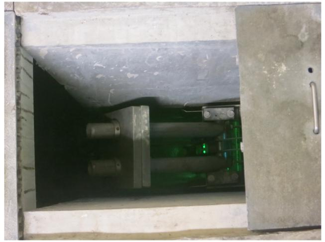
This is the UV disinfection channel. After the tertiary filtration by the dual media filter, effluent is disinfected by UV light. The reclaimed water can be used after that.
