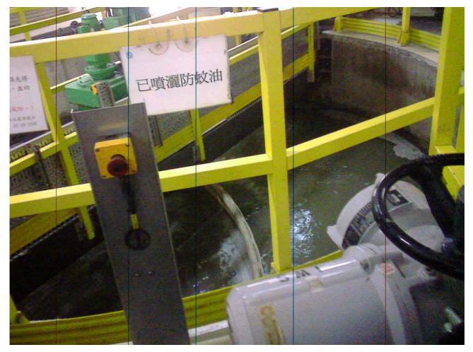
Device in the photo is the grease separator which refers to the inlet works and is used to remove the grease in the sewage to protect the downstream treatment process.
