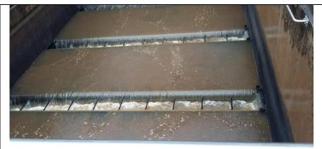
This is a sedimentation tank. After sedimentation, the water will be clean and go to the filtration tank.
