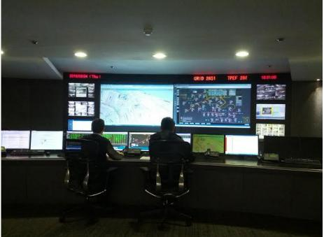
This is the control center of Towngas. The technicians can check the status of the gas delivery pipe via the system and make the necessary adjustments.
